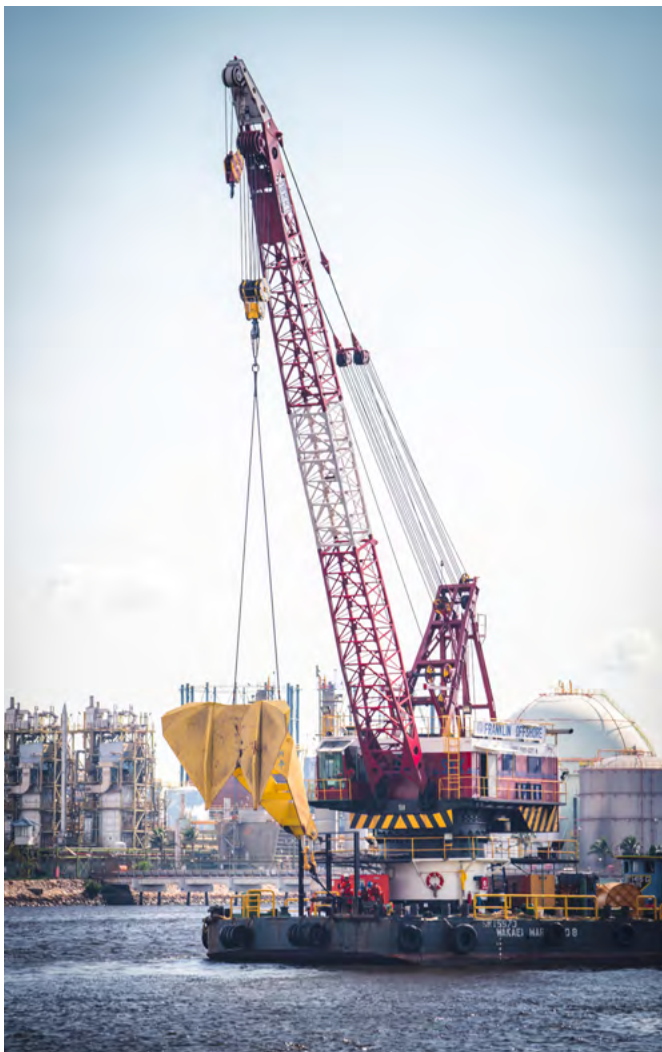
Wakaei Maru No. 8 100 Tonne Crane Barge
